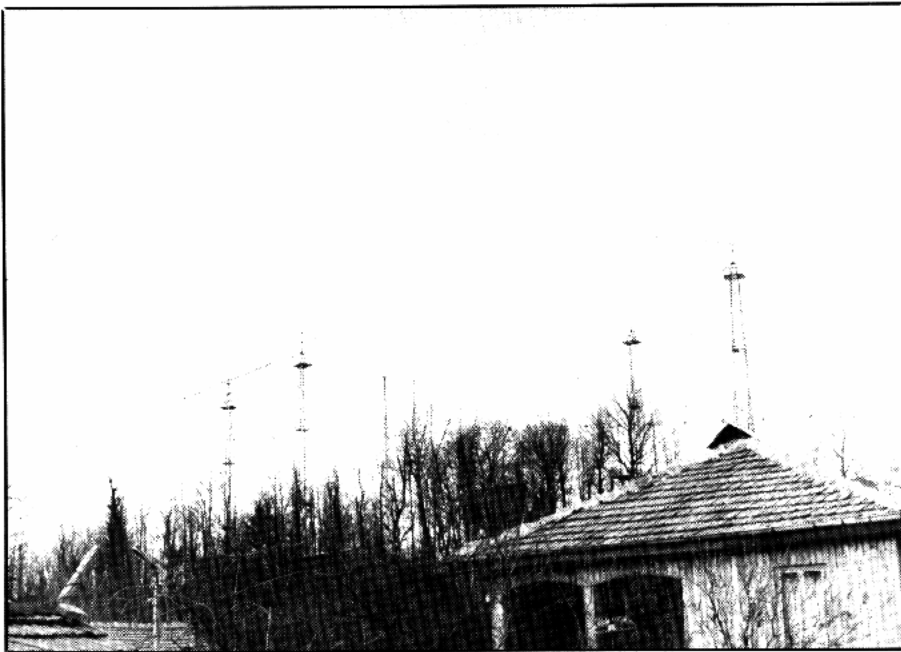
The boys at LZ9A, also LZ2KTS, sported this fine set of antennas—6 elements each on 10, 15, and 20, and 4 elements on 40.
